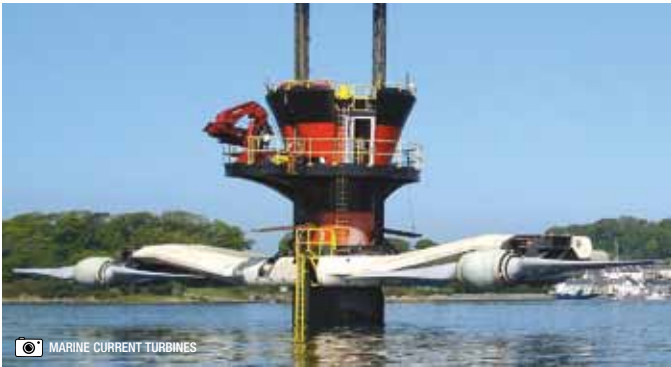
Marine Current Turbines' tidal turbine is seen out of the water for maintenance in Strangford Lough, Northern Ireland.
